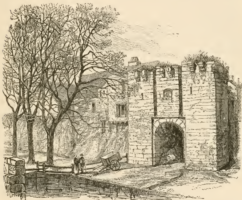
Part of Walls and Gateway, La Guérande.
